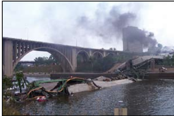
Figure 1.1: Collapsed I-35W Bridge.
