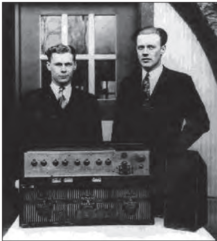
Figure 1-1: Detroit Police Department Station KOP (1928)
